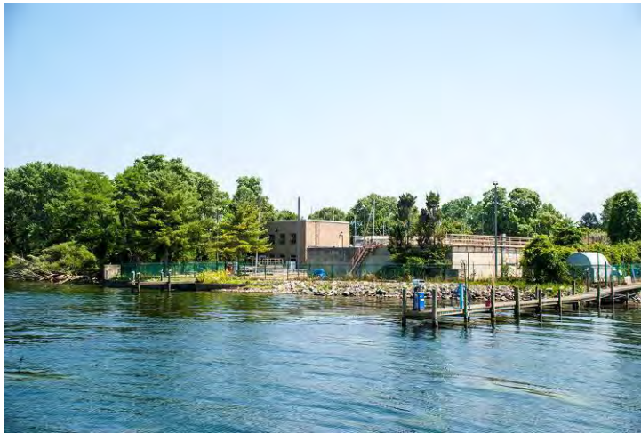
The wastewater treatment plant lies right on the lakefront.
