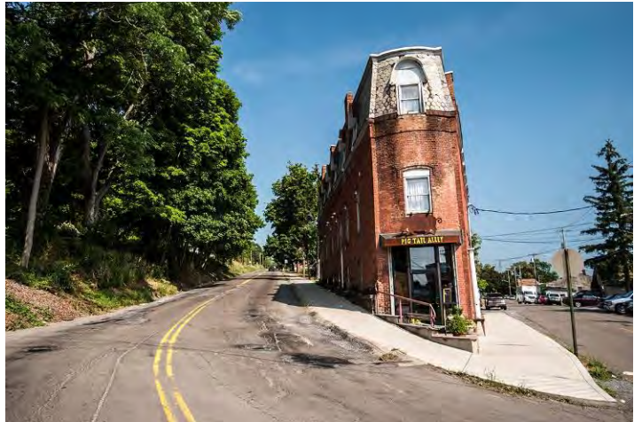
The Flatiron Building was an important landmark in races.
