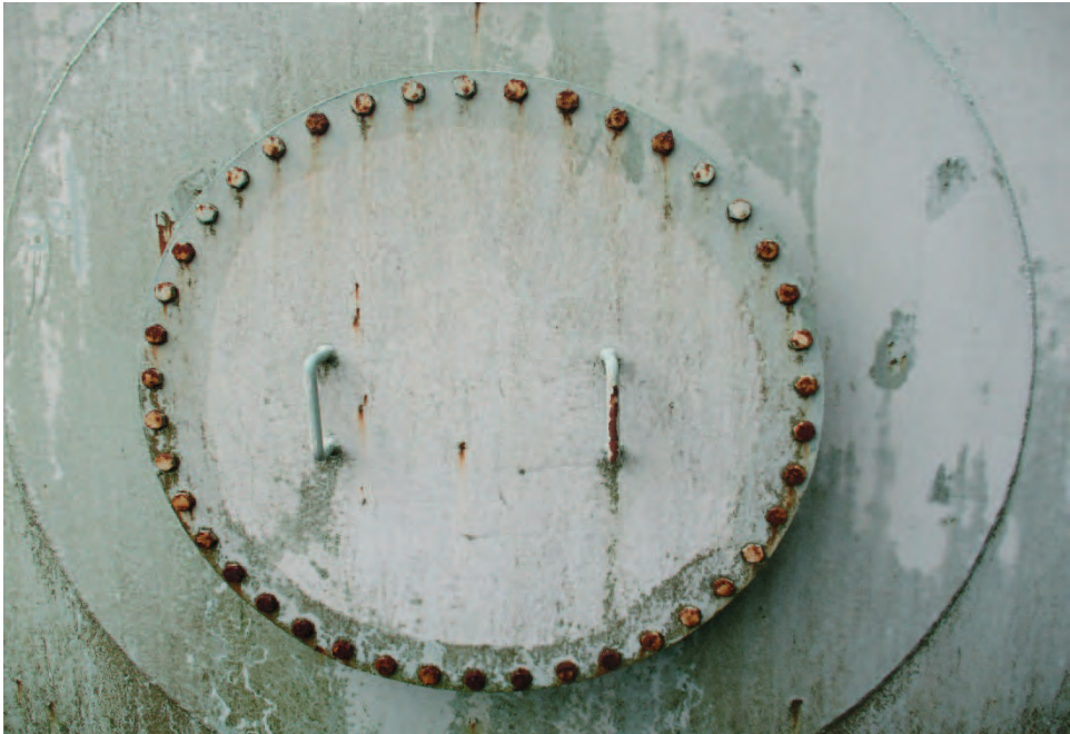
Exterior Side Shell Access
