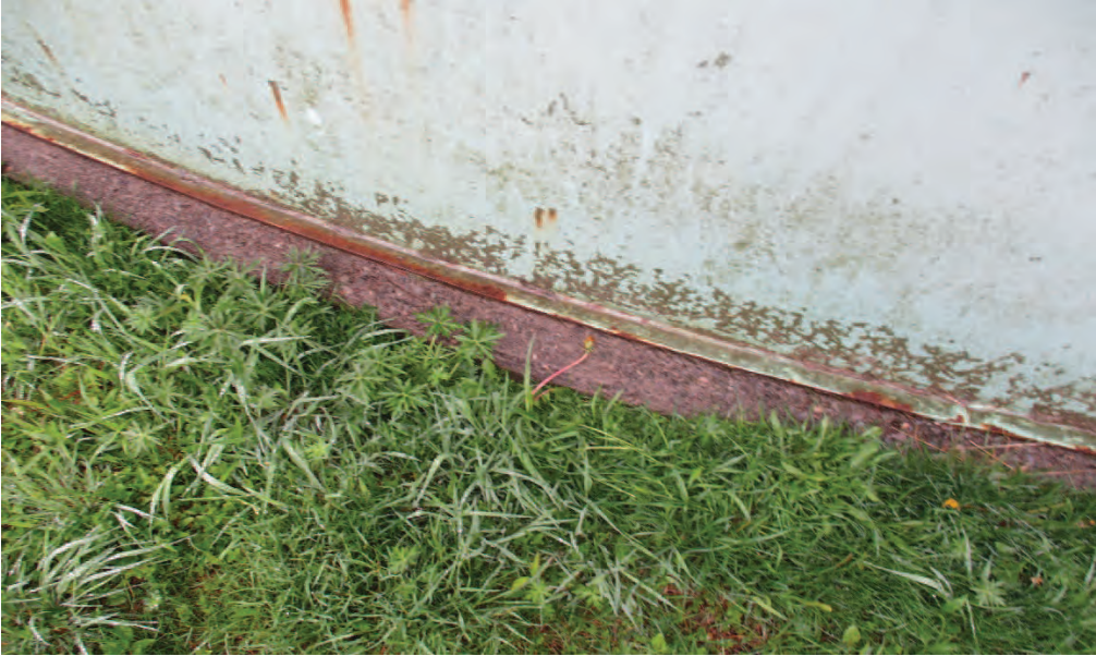
Exterior Tank Base
