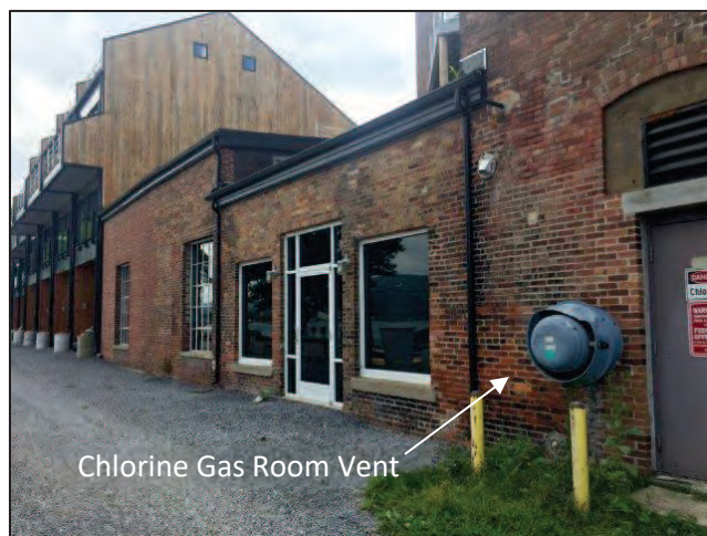
Figure 1: Raw Water Chlorine Gas Room & Apartments
