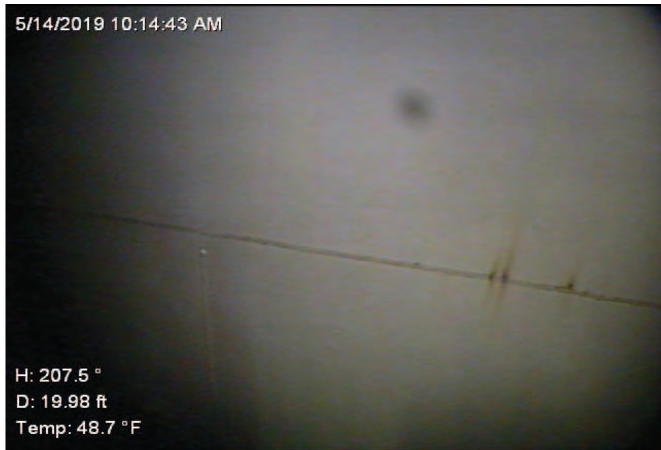
Interior Side Walls
