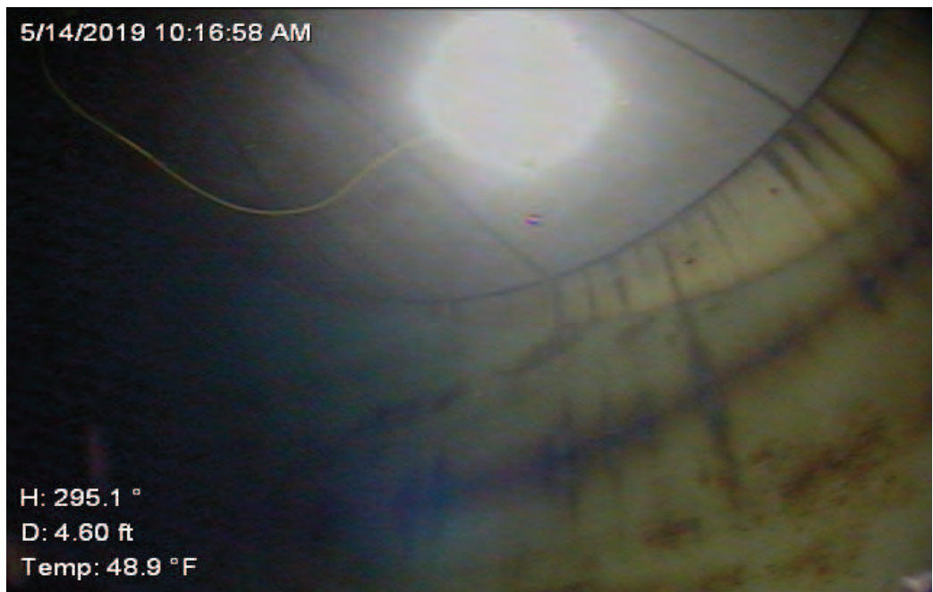
Interior Side Walls
