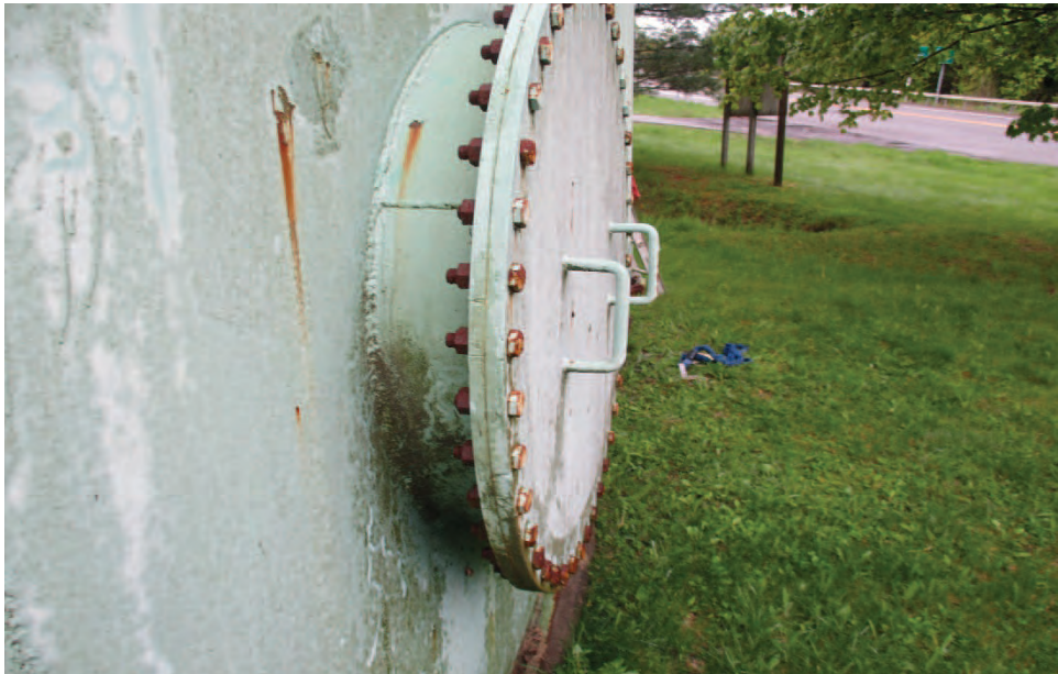
Side Shell Access
