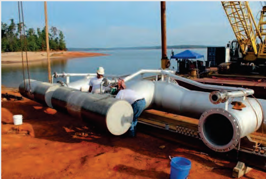
JOHNSON SCREENS® Passive Intake Installation: Drinking Water Plant in South Carolina, USA
