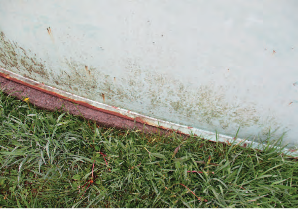
Exterior Tank Base
