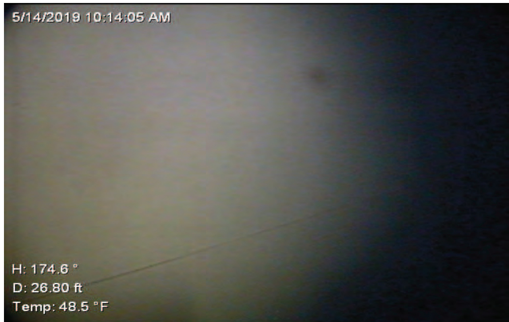
Interior Side Walls
