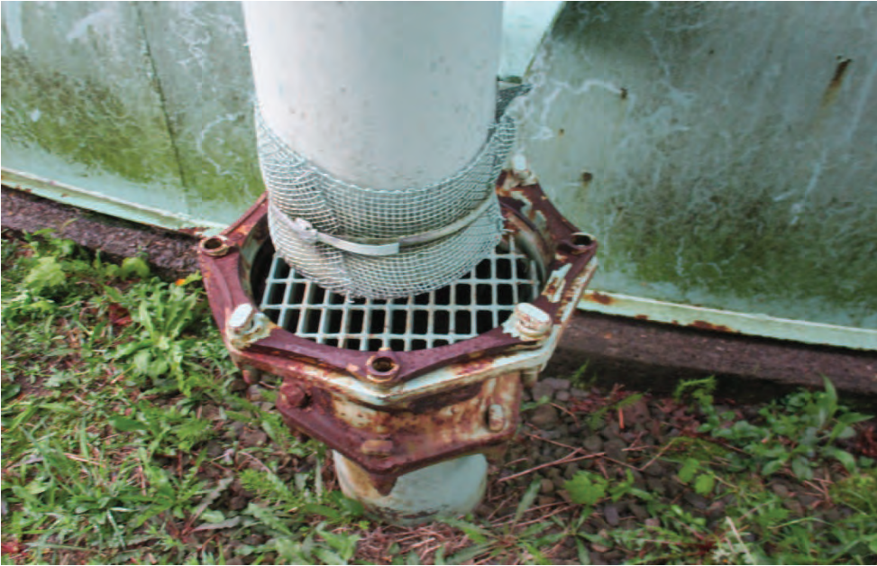
Exterior Overflow Screen
