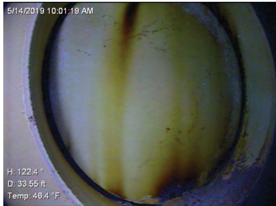
Interior Side Shell Access
