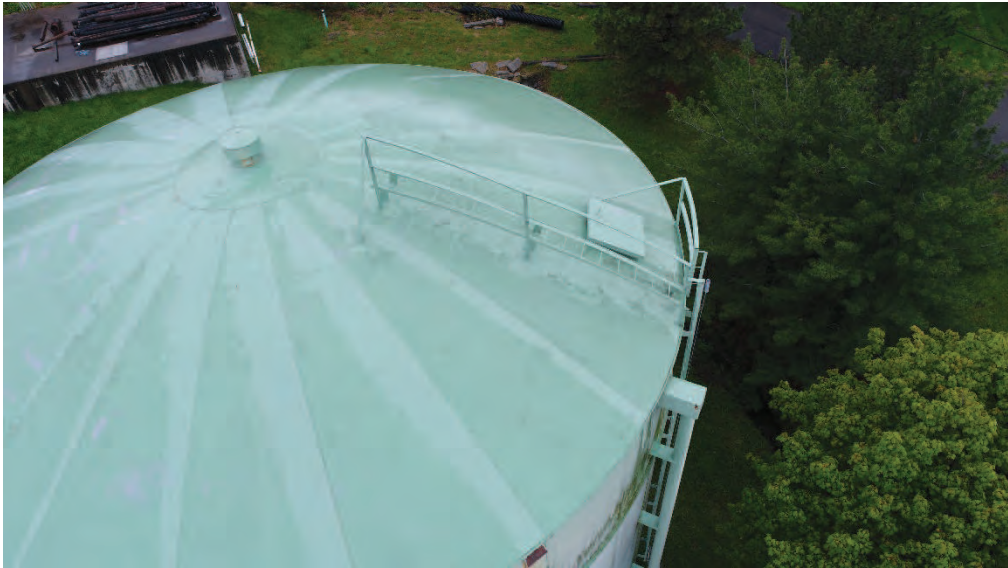
Exterior Drone Ceiling Photos
