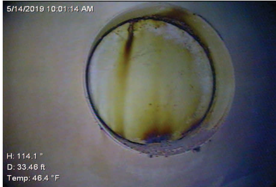
Interior Side Shell Access
